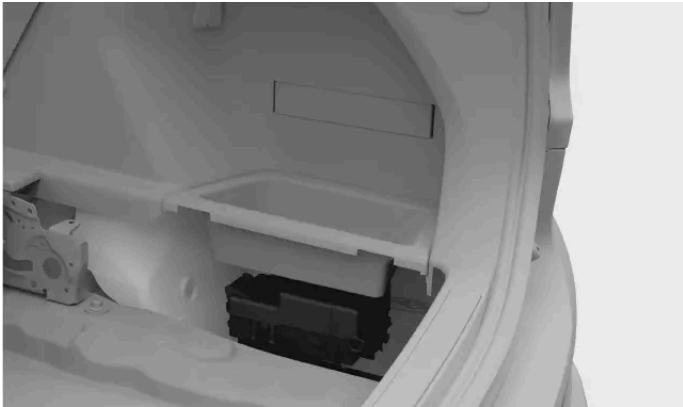
Fuse box location
