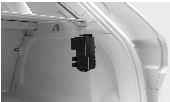
Fuse box location
