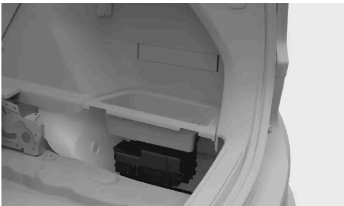
Fuse box location
