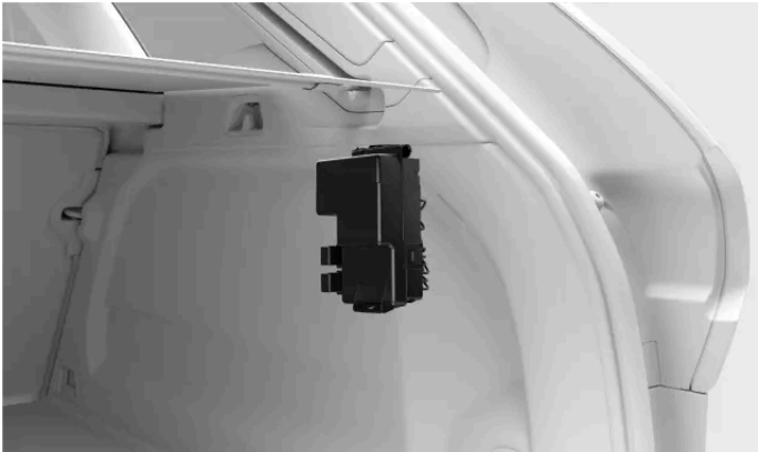
Fuse box location
